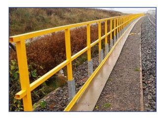
Posts are pre-routed to accept continuous rails, eliminating the need for extra pieces to connect rails to posts.
