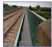
Fibregrid fabricated the underbridge walkway sections in 3mtr units for ease of transportation and installation at site.
