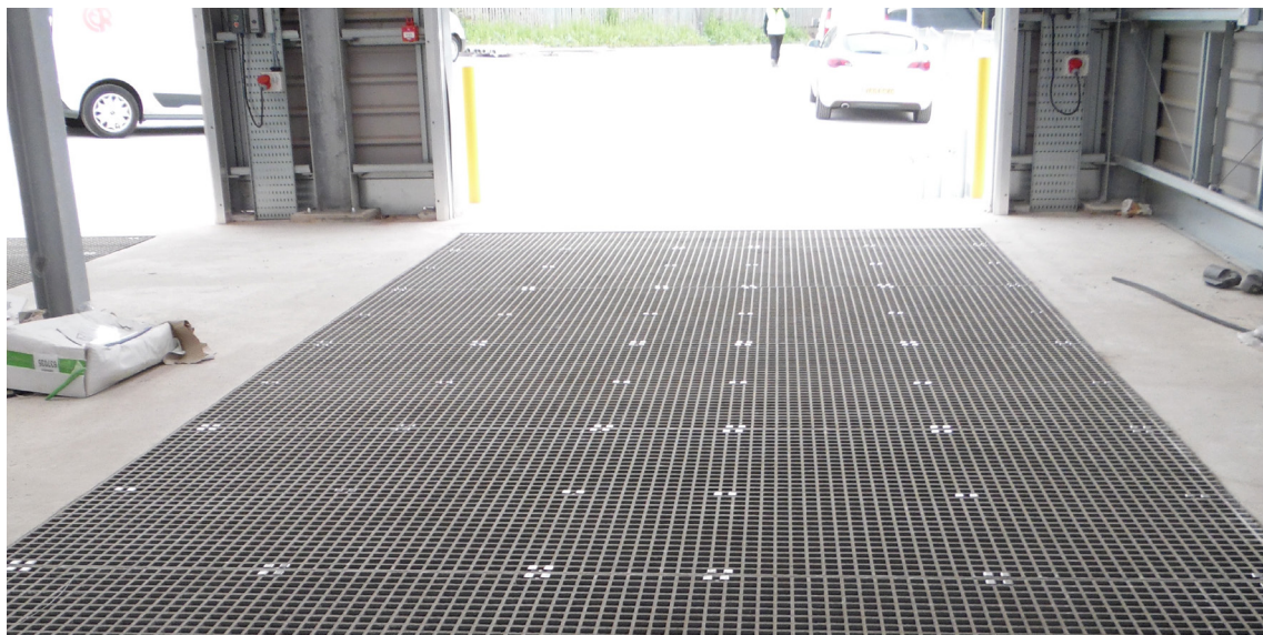
Bespoke lift out sump area
