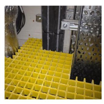
Service risers, also known as decking risers, or shaft risers are often used to provide a safe working environment, during construction, refurbishment or demolition. Our GRP Heavy Duty Embedded Grit Top Grating is a cost effective, anti slip alternative to traditional steel grating and it was successfully installed by Como, a Mace contractor, for one of their high rise building projects.
